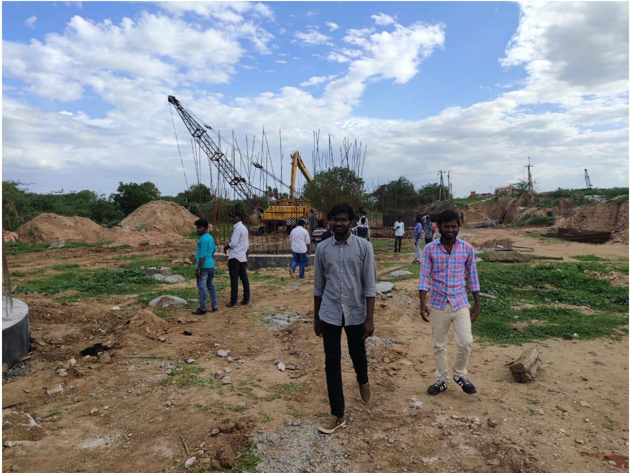
Students observing various components of Bridge
